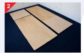
Place your other 1m x 1m and 2m x 1m Harlequin Liberty® sprung floor panels onto your sub-floor, so that they are in a brickwork layout. Push the panels against the other panels and join them together using the locking tool.
