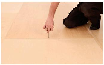
To fit around obstructions such as pillars, cut the panels to size allowing an expansion gap of 10mm and stick extra pads on the underside of the cut edges using double-sided tape before latching in place.
