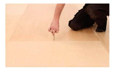
To fit around obstructions such as pillars, cut the panels to size allowing an expansion gap of 10mm and stick extra pads on the underside of the cut edges using double-sided tape before latching in place.
