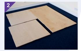
Place your other 1m x 1m Harlequin Liberty<sup>®</sup> sprung floor panel onto your sub-floor and push it into place. Join this panel to the others using the locking tool.
